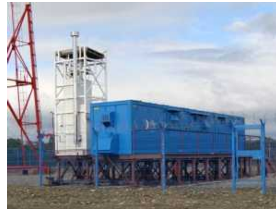
Steam turbine generators ORMAT
