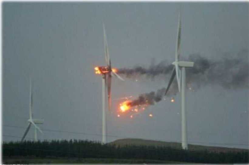
Ignition of electrical generator
