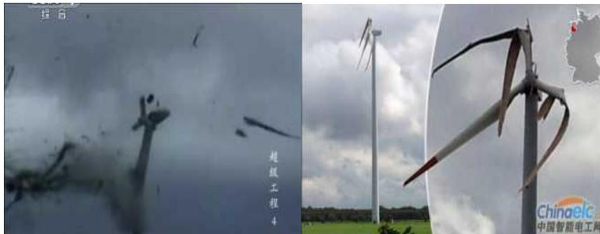
Figure 1 failure mode after the typhoon
